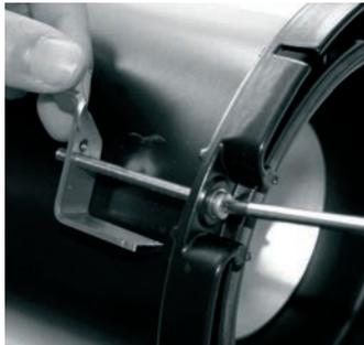
Mount the bracket which corresponds to the thickness of the false ceiling. Attach the safety cable to the ceiling (Pathe C/R-S4 and C/R-S5 versions).
